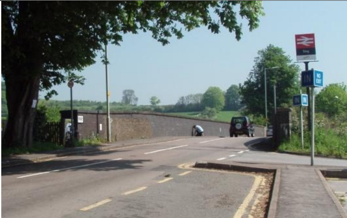
Figure 2 – Tring Station Bridge from the west
