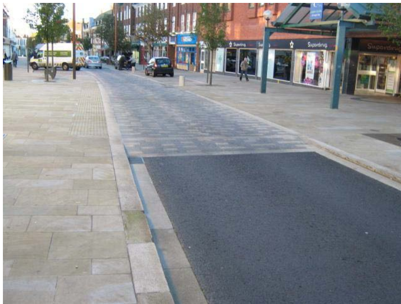
Figure 7 – Example of well constructed carriageway blocks from Road’s in Hertfordshire Design Guidance
