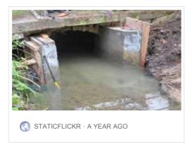
Concrete walls installed, just removing the wooden shuttering
