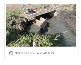
Wooden shuttering being installed to cast the concrete bridge support
