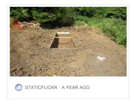
One of the vehcile bridge foundations waiting to be filled with concrete
