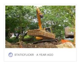
Decking boards for vehicle bridge being unloaded
