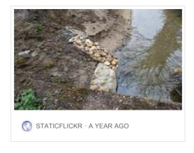
Behind gabion backfilled; stone detail on top of concrete to match gabion
