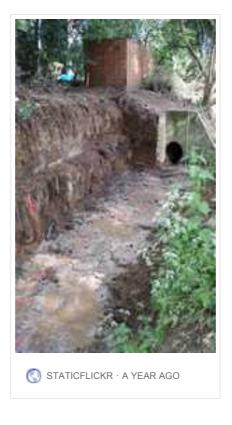
Headwall has been cut back and all concrete removed
