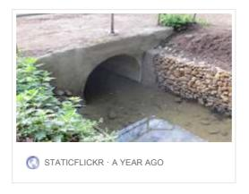
Headwall on downstream side also repaired
