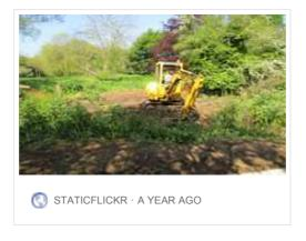
Digger reprofiling the bank edge once the culvert had been removed
