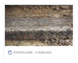
Geogrid being installed to strengthen the bank
