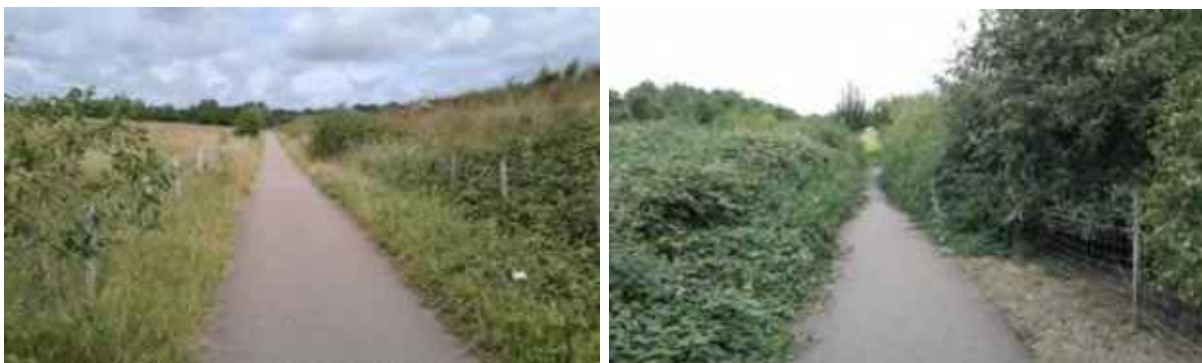
Figure 8. The section managed by Tarmac Ltd is generally more open, but its width is reduced in places by tall and encroaching vegetation.
