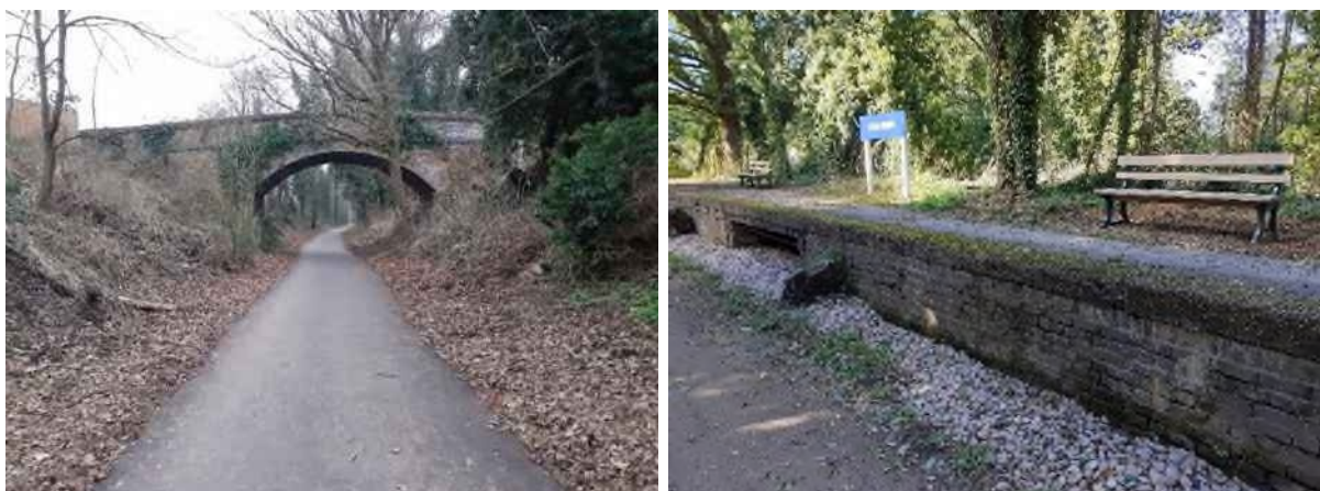
Figure 2. Hertingfordbury Park Bridge and Cole Green station platform.
